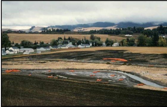
CHANNEL AFTER EARTH WORK
