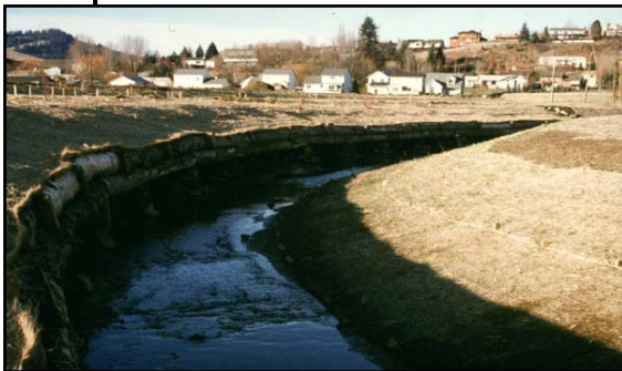
LOG CRIB REVETMENT
